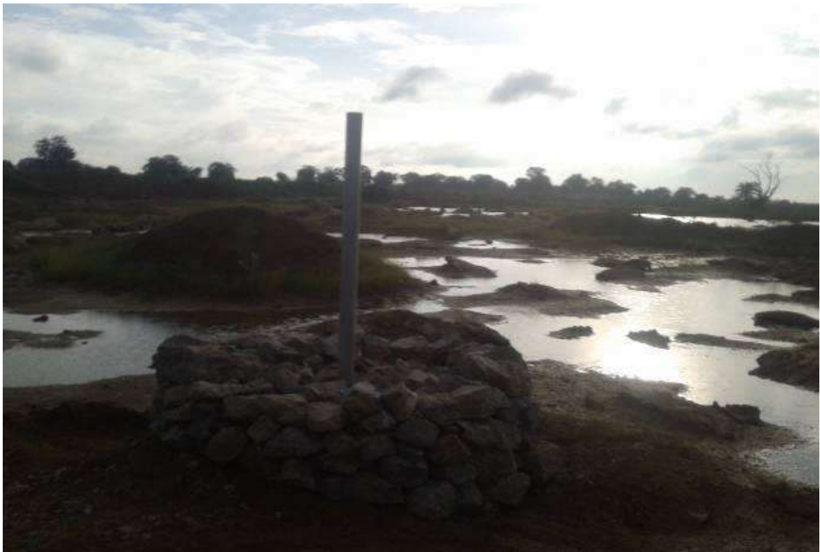
Figure 4 Recharge Well No-4
