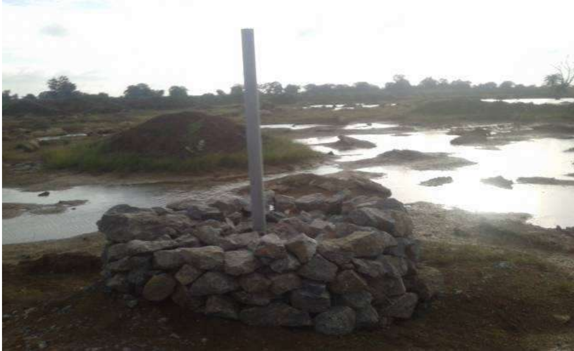
Figure 3 Recharge Well No-3
