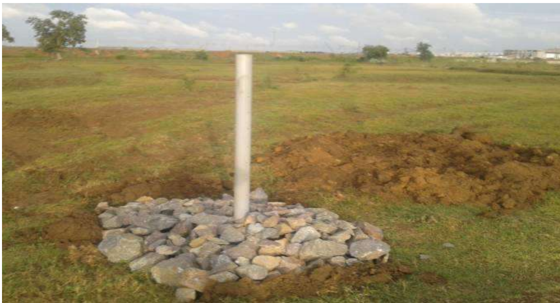
Figure 2 Recharge Well No 2
